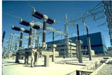
Figure 55: Tungsten based switch (left) used at SF 6 circuit breaker (right) (Böning).
